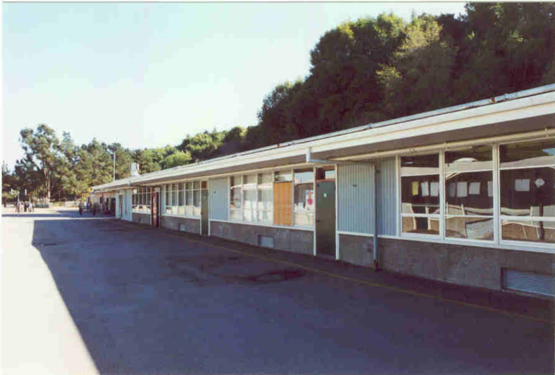
Figure 4: East Elevation of Main Classroom Building (portables behind)
