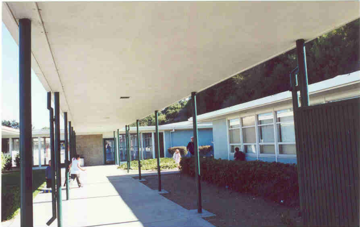
Figure 6: Covered Walkway between Multi-purpose Room and Main Classroom Buildings
