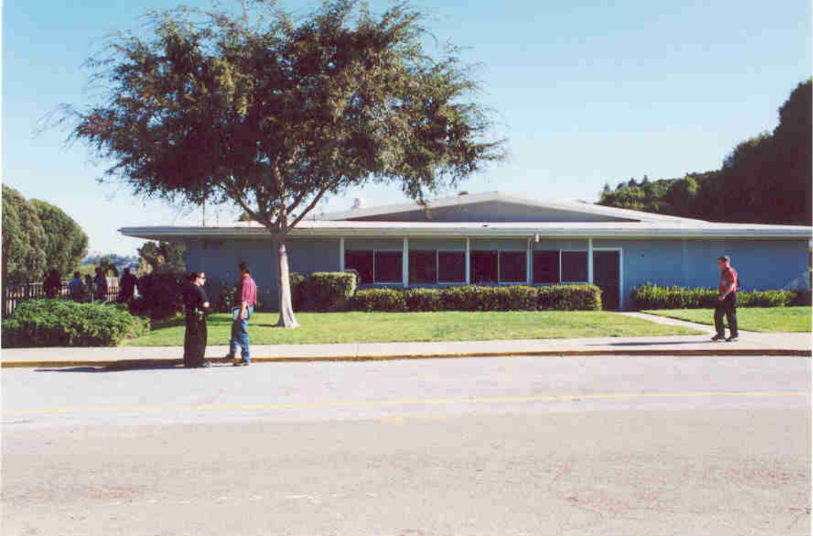
Figure 2: North-west Elevation Looking at School Offices
